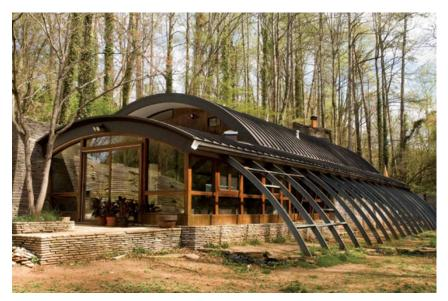
A third corrugated metal roof was installed over the second years later during building renovations. Other roofing materials were considered as replacements, but later discarded since the original roof was welded to the Quonset hut beams.
