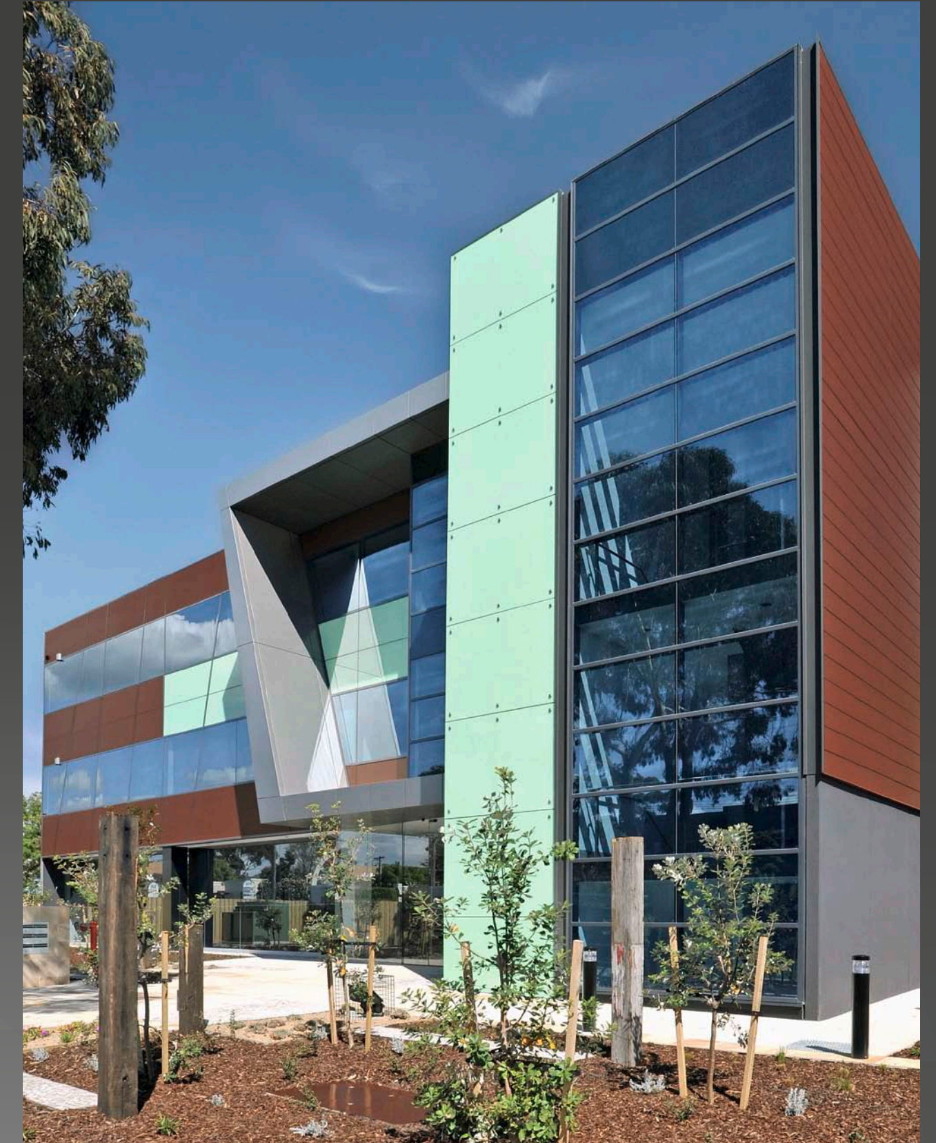
Mainstreet Mornington, Australia | Material: ALUCOBOND® Wood Design Redwood
