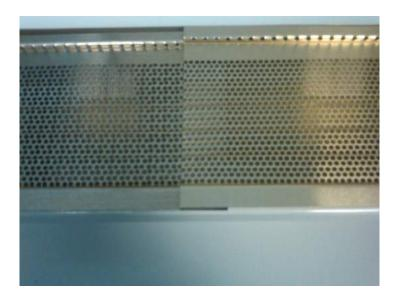
4. Install 3 zip screws on front lip of each MicroGuard screen. One screw should be on each end through overlap (where there is one) and one in the middle.
