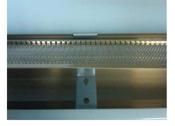
2. Place front of MicroGuard (Z bend) on top lip of gutter.
