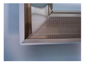
6. At end cap, cut the tabs to approximately 1" back in order to fold the end down into the gutter and behind the end cap.
